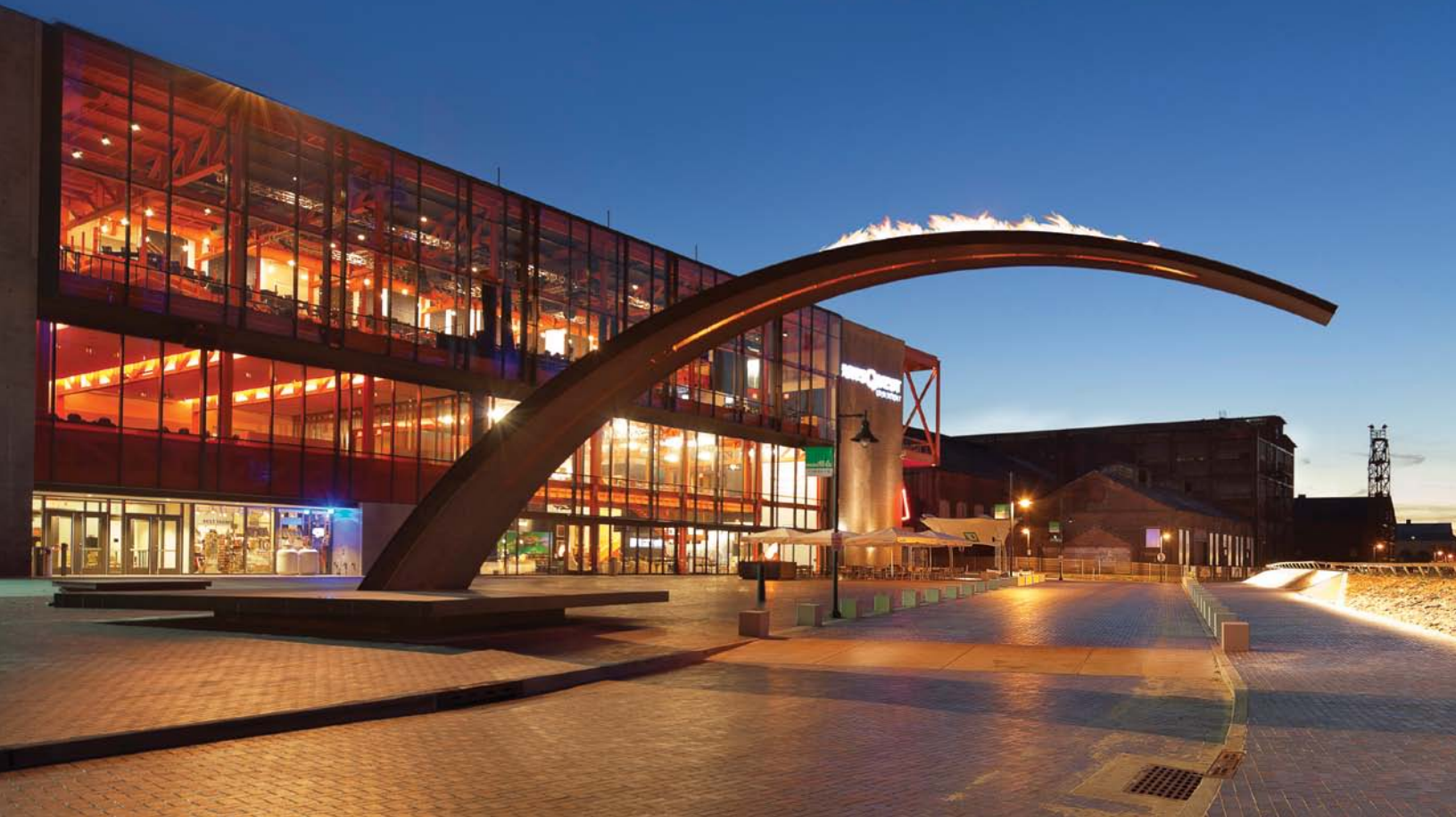
The Bridge , designed by Elena Colombo, was funded by an NEA MICD25 grant. PHOTO BY PAUL WARCHO
